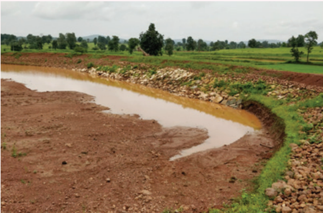
Figure 17 Water harvesting ponds to collect runoff water from fields
