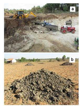
Figure 1. (a) Desilting of water harvesting tanks using machine (b) Tank silt
